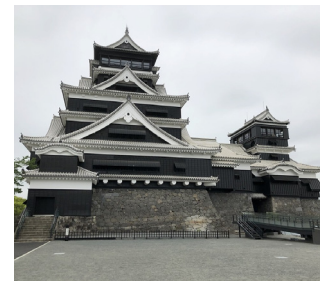
Kumamoto Castle (Under restoration)
