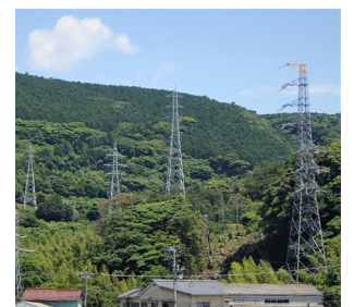
TEPCO Power Grid, Incorporated Inatori Power Line (66,000 volts)
