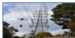
Replacing the Koto Liaison Line Insulator
